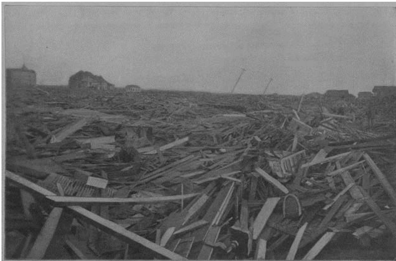
GENERAL VIEW ALONG THE GALVESTON BEACH AFTER THE FLOOD
