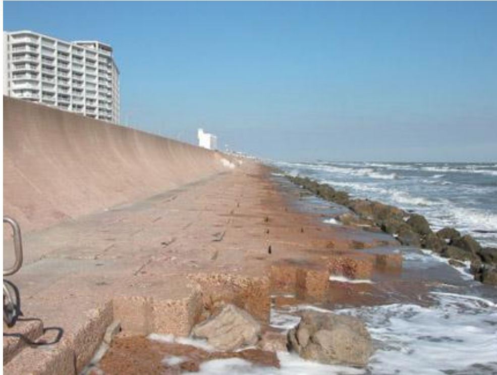
Galveston Sea Wall constructed in 1902
