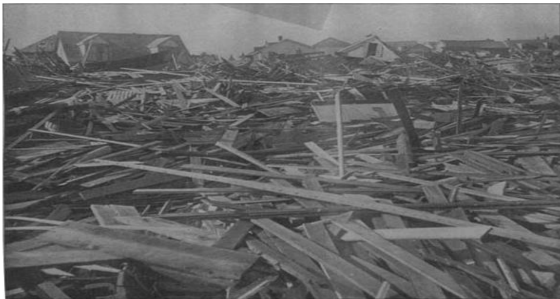
GREAT MASS OF DEBRIS ON THE WEST END—GALVESTON
