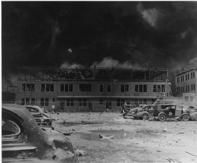
Shattered and burning remains of the Monsanto plant.
